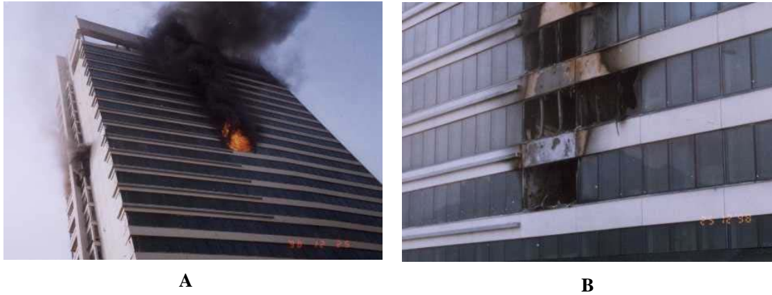
Figure 2: (A) Fire occurs at the 14 th floor. The building is under construction and sprinkler system is not in operation. The room of fire origin stores mattresses and other combustible materials. (B) External wall conditions after fire.
