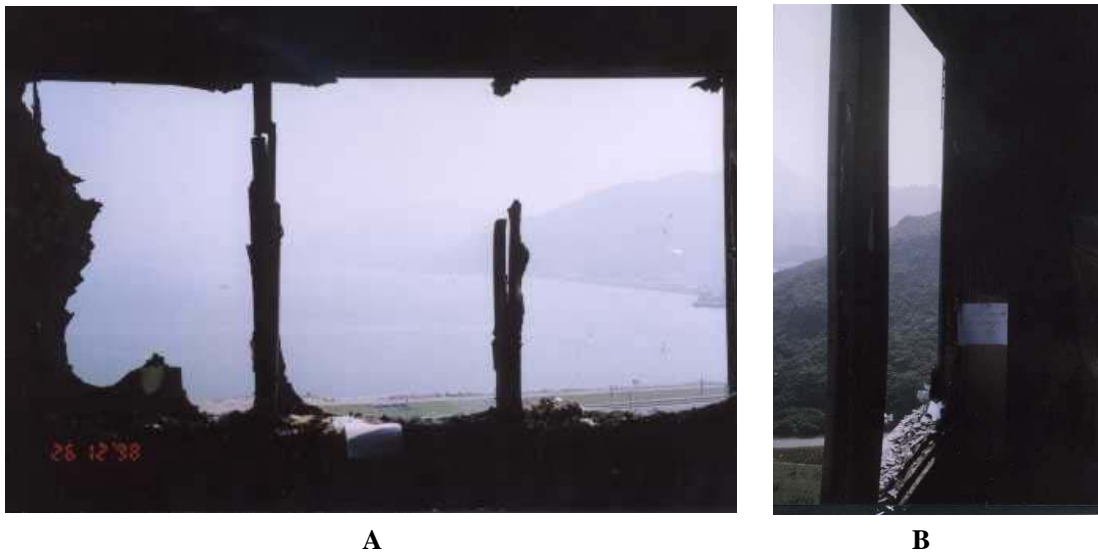
Figure 3: (A) Internal view of window of the room at the 16 th floor. (B) Internal view of window of the room at the 15 th floor.
