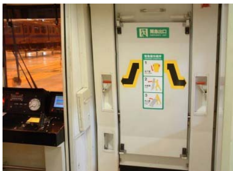
Figure 20. The exterior air release vent valve of the Taipei MRT car
