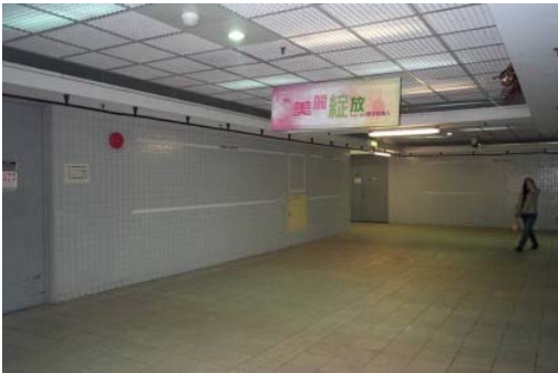
Figure 9. The leaky cable of the underground station in Taipei MRT
