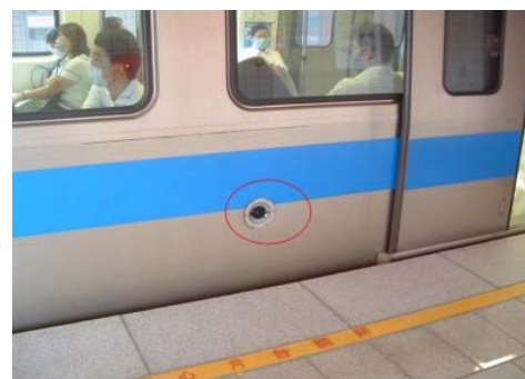
Figure 21. The Escape ramp of the Taipei MRT car
