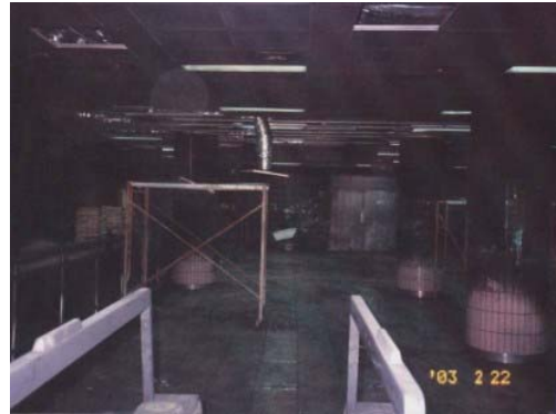
Figure 2. The underground second floor of the concourse level in the subway Jungangon Station
