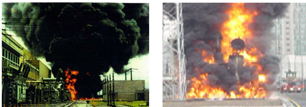
Fig.2 Fire incidents in transformers
