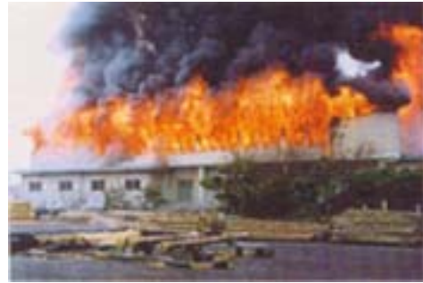
Photo1. Picture record of the fire (from the west side)
