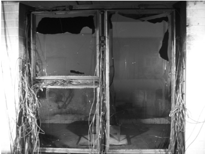
FIGURE 15. Breakage and fallout of float glass
