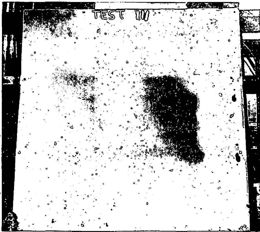
FIG.9. APPEARANCE OF CEILING AFTER TEST 3
