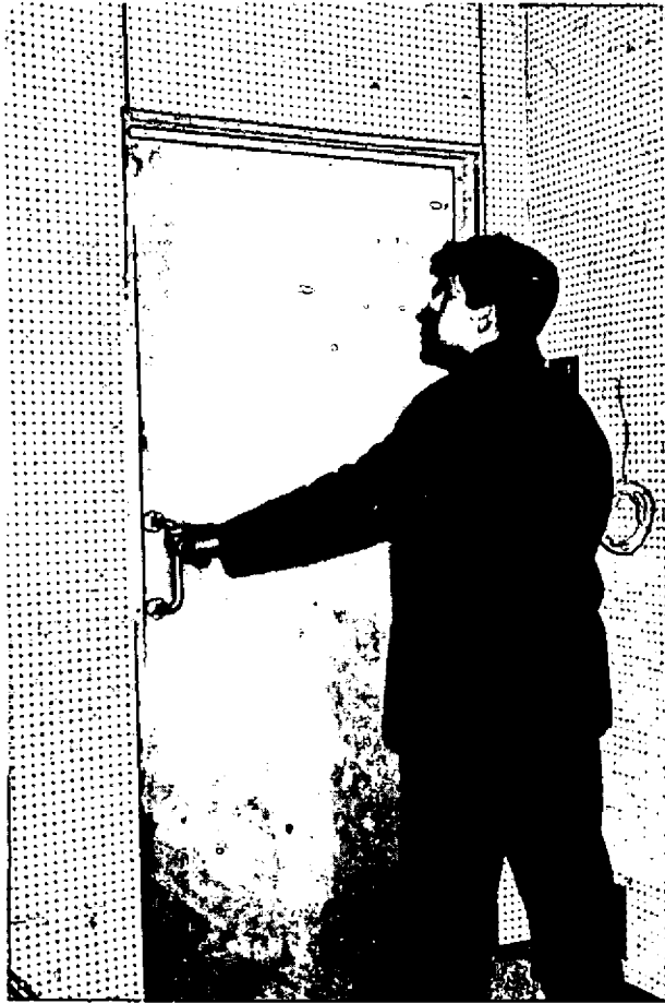
FIG. 9 DOOR No. 1 ON GROUND FLOOR
