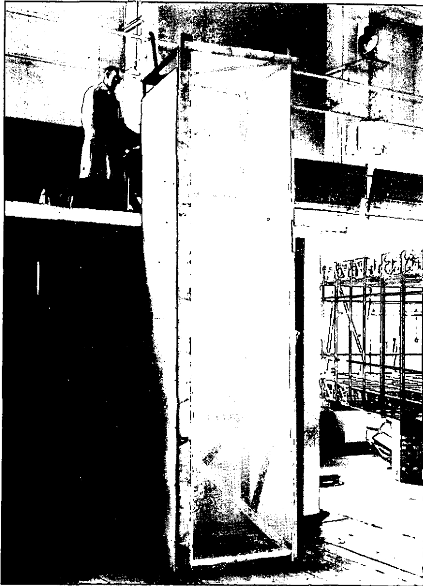
APPARATUS FOR MEASURING THE RETENTION OF FOAM BEHIND A NET
