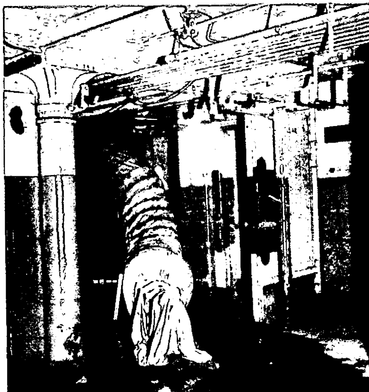
FIG. 4. INTRODUCTION OF DUCT INTO BASEMENT 3.1 m (10ft) BELOW GROUND
