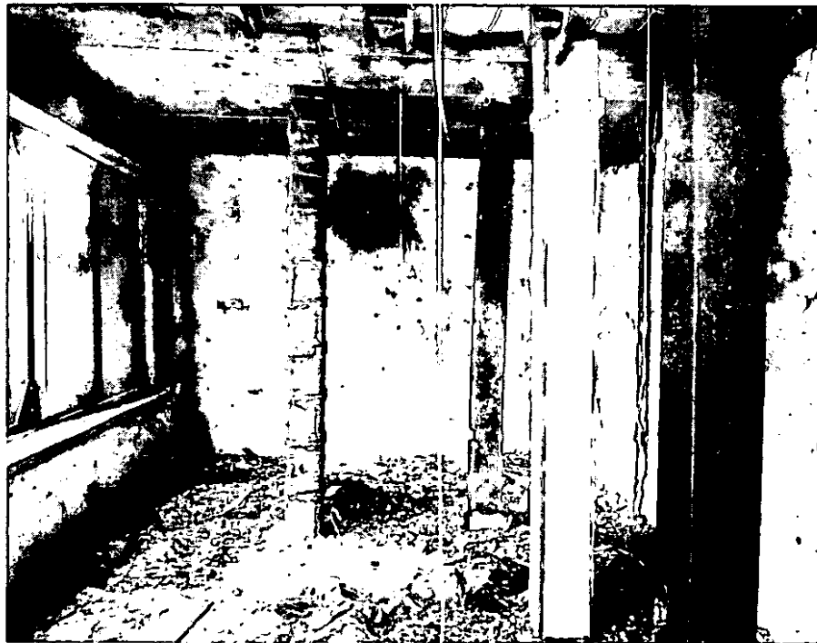
PLATE 4. TEST COMPARTMENT AFTER TEST SHOWING THE COMPLETE BURNOUT
