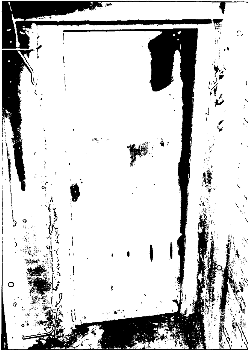
PLATE 1. CONDITION OF DOOR OF FIRE CHAMBER AT END OF PRESSURIZED FIRE TEST
