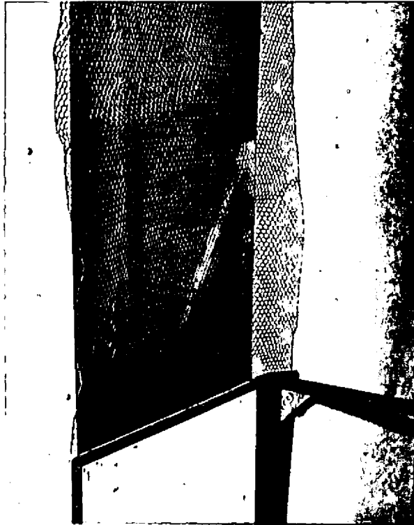
WIRE MESH PANEL IN ONE SIDE OF FOAM ENCLOSURE
