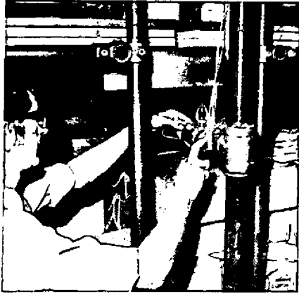
Sprinkler and baffle PLATE 1
