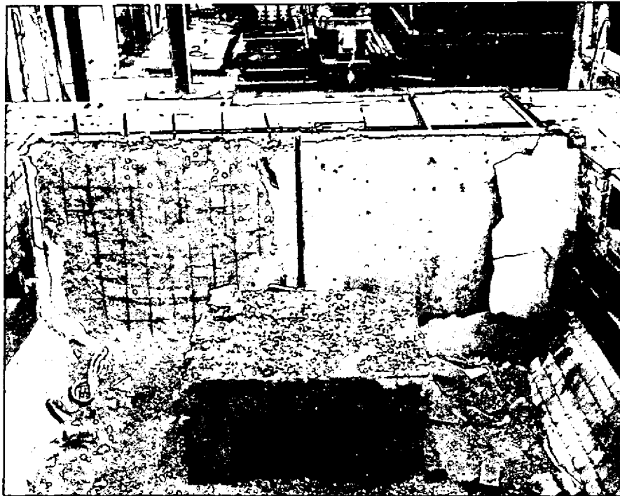
FIG. 18. APPEARANCE OF FACE OF WALL UNITS EXPOSED TO FIRE AFTER TEST (CONSTRUCTION 1 ON LEFT)
