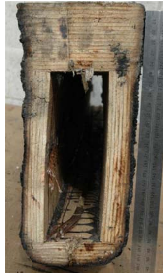
Fig 2. A section of timber box-beam after fire exposure. [4]
