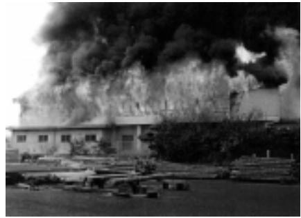
PHOTO 1 Fire-damaged building in flames
