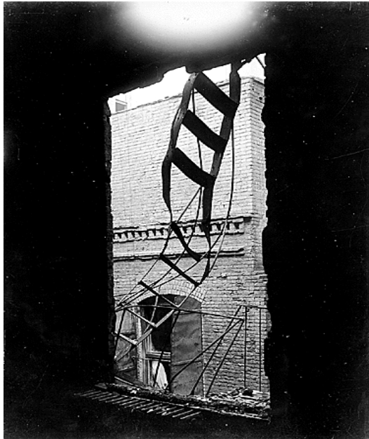
Figure 3. Triangle Shirtwaist fire escape ladder. Reproduced with permission from the Franklin D. Roosevelt Presidential Library.
