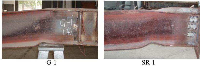
Fig. 11. Local flange buckling.
