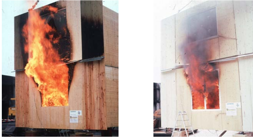
Fig. 5. Fire development 7 minutes after fire ignition; left: lower module with combustible linings (fire test BÜ bb), right: lower module with non combustible linings (fire test BÜ nbb).
