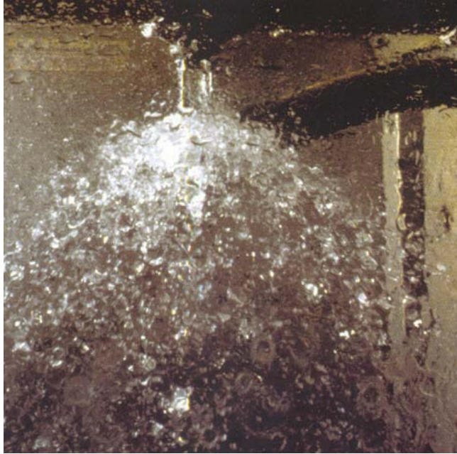
Fig. 2. Example of the functional test of the sprinklers.
