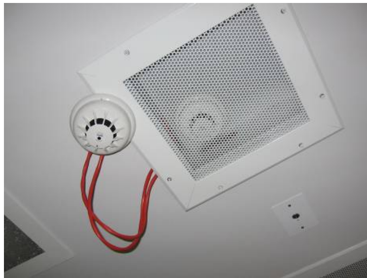
Fig. 4. Recessed detector with surface mounted detector for testing.
