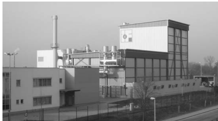
Fig. 8. Test facilities in Heyrothsberge (maximum room size: 5100 m 3 (255 m 2 ), 3000 m 3 (300 m 2 ), 500 m 3 (50 m 2 ), 250 m 3 (25 m 2 ); tunnel: 6.5 m 2 x 30 m).
