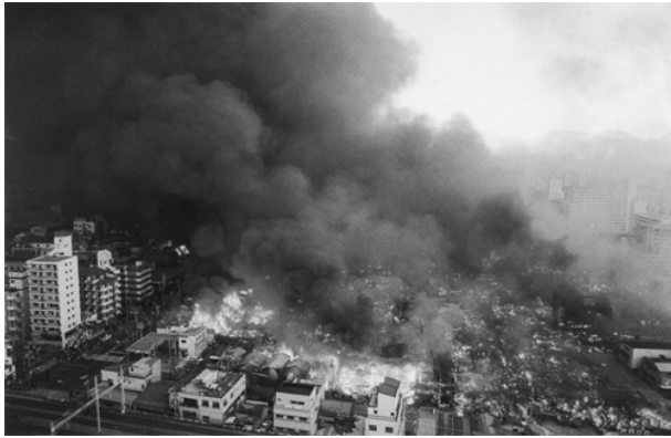
Fig. 1. Fires followed Kobe Earthquake 1995 [11].
